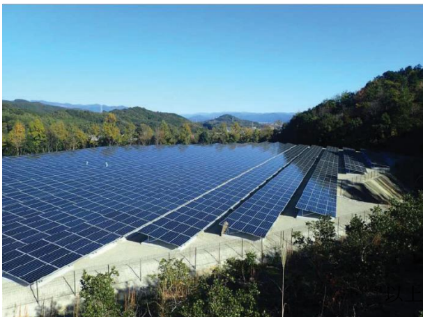
Kochi Soler Power Plant Details
